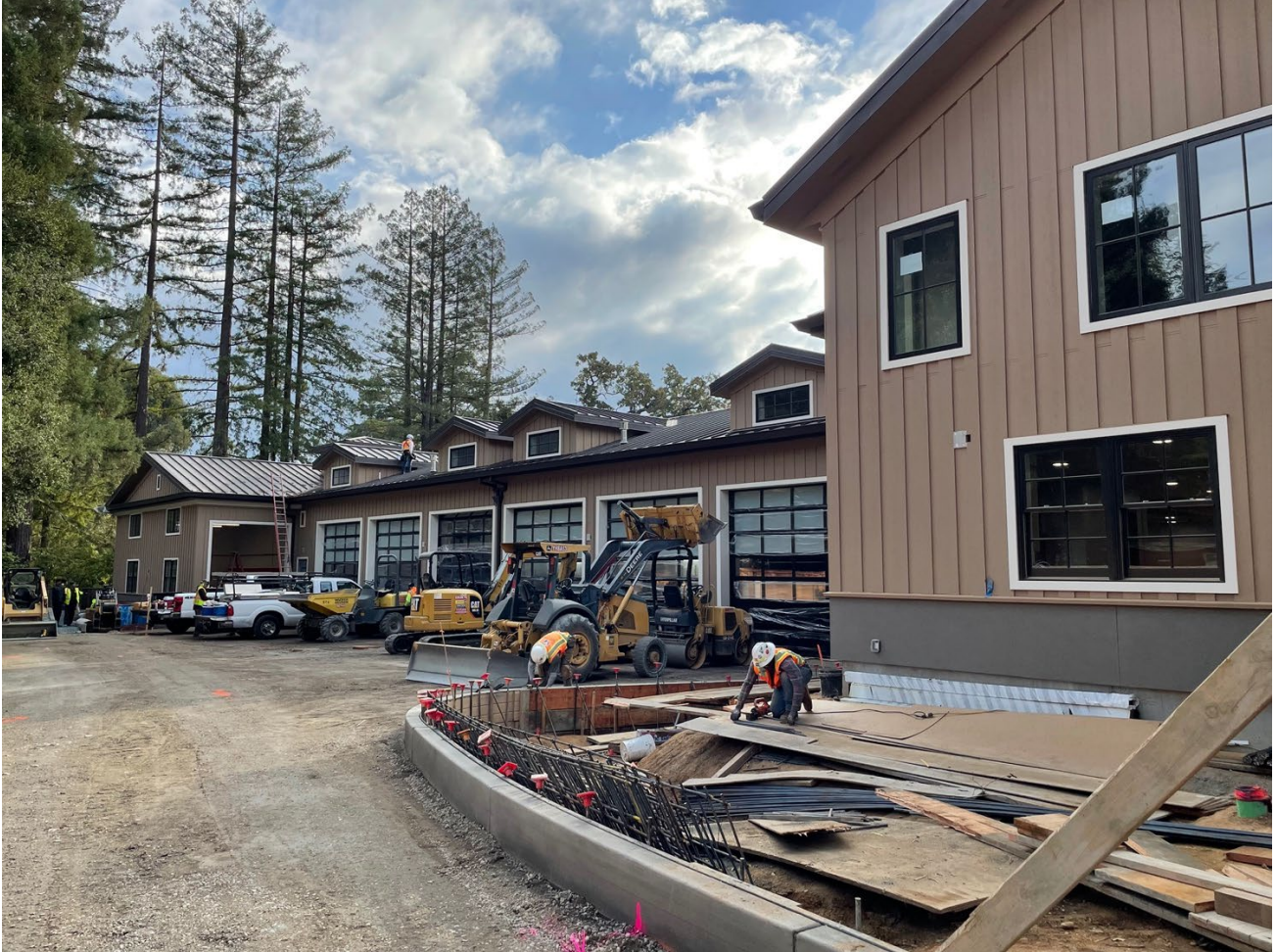
(East side of the station rear side apparatus Bay and shop)
