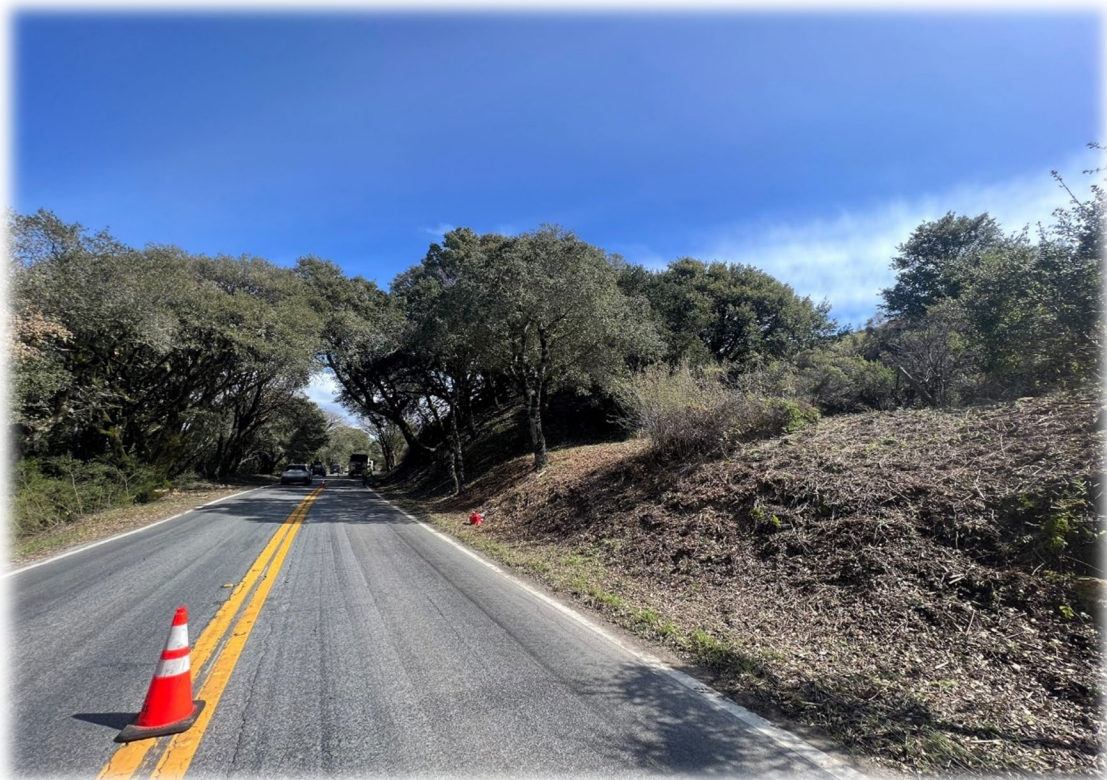
Figure 2 Skyline Grant Project - After Shot
