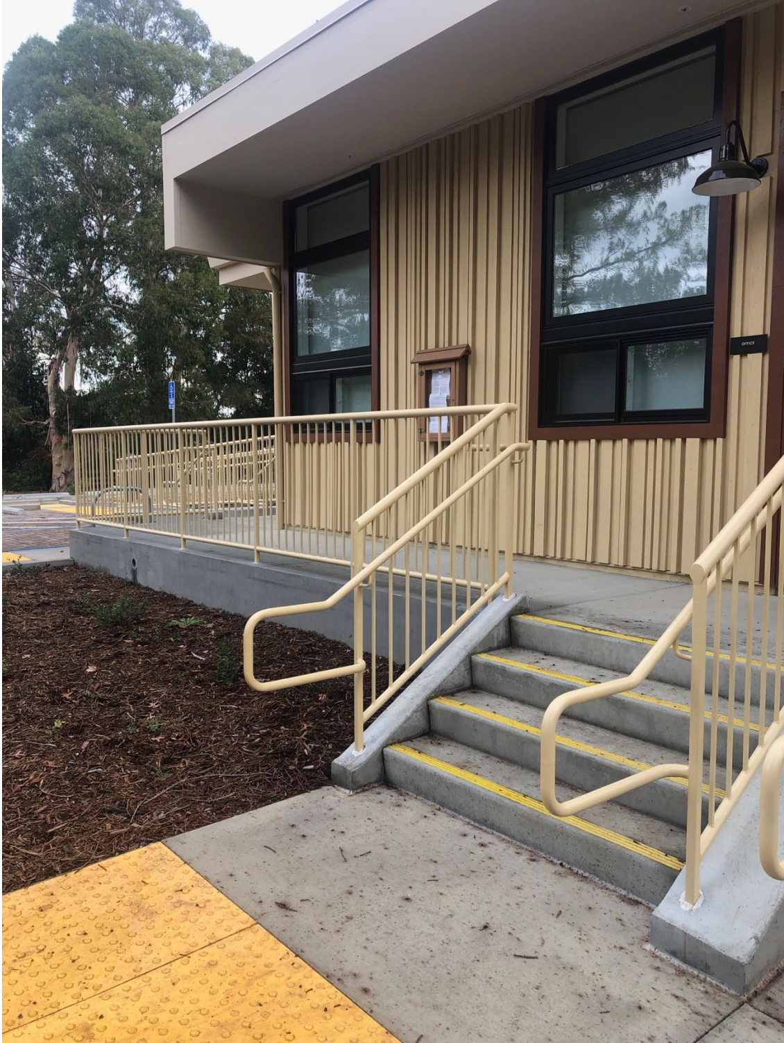
(Outside rails completed and painted front walkway station 8)
