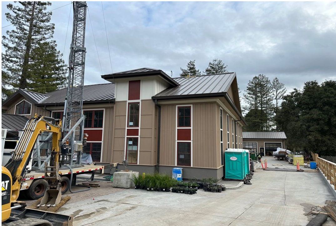
West driveway concrete complete
