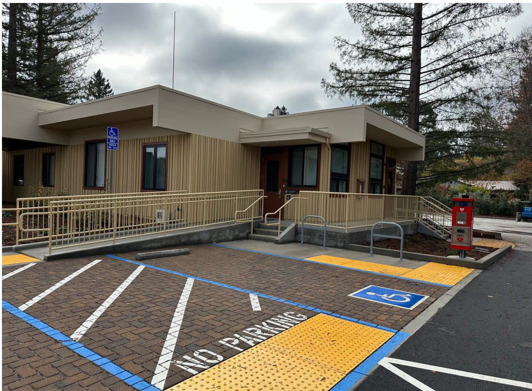
North Driveway, painting ADA strips and pavers complete. AED Unit installed.
