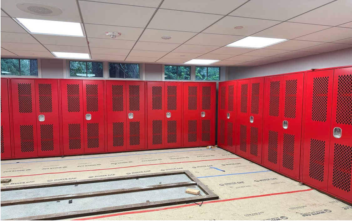
Turnout locker installation underway
