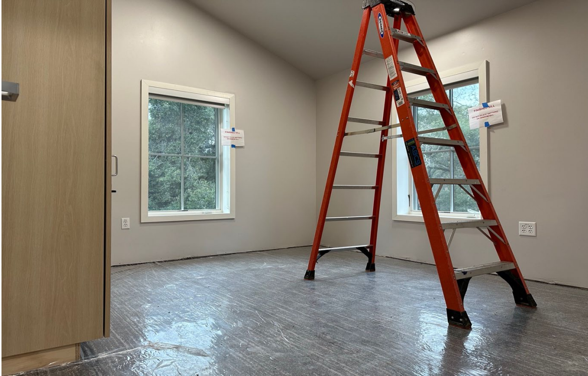
Bedrooms complete with casework, paint, trim window coverings and carpet installed
