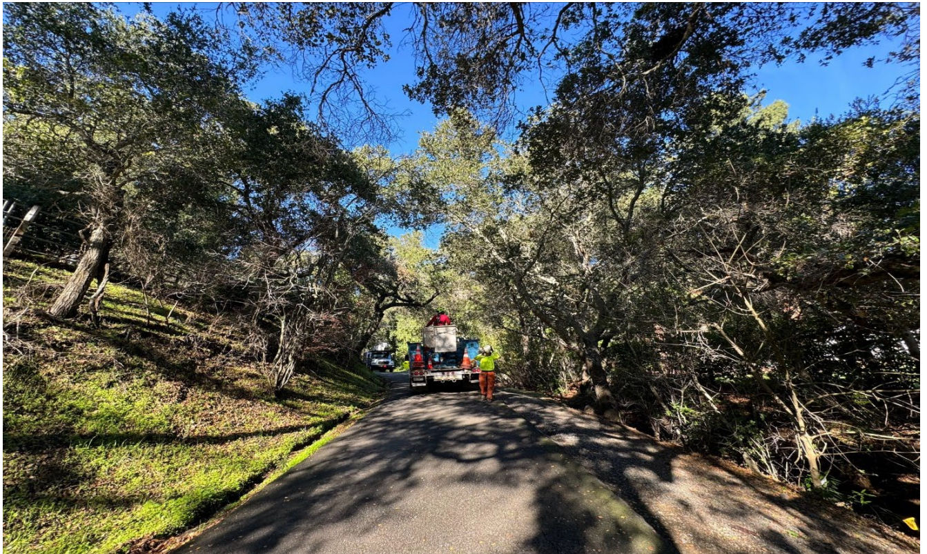
Glencrag Road- Before Shot
