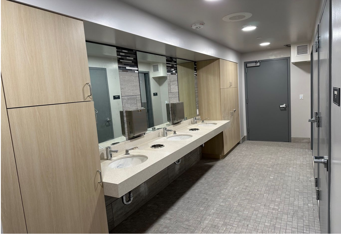
Downstairs bathroom complete
