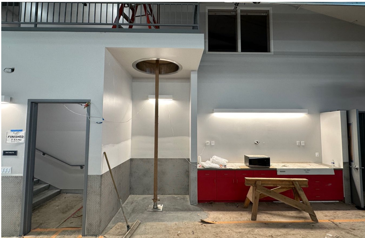
Fire pole installation underway
