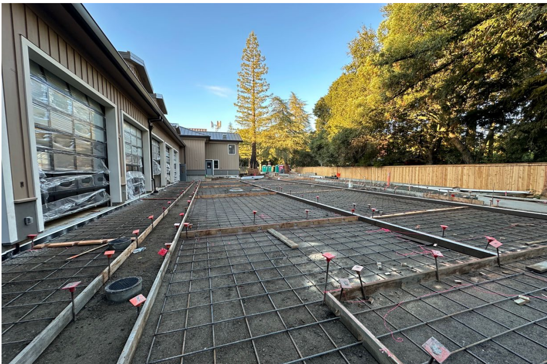
East driveway rebar and forms
