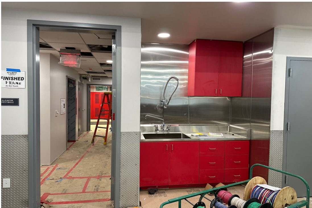
Casework and stainless steel in apparatus bay complete
