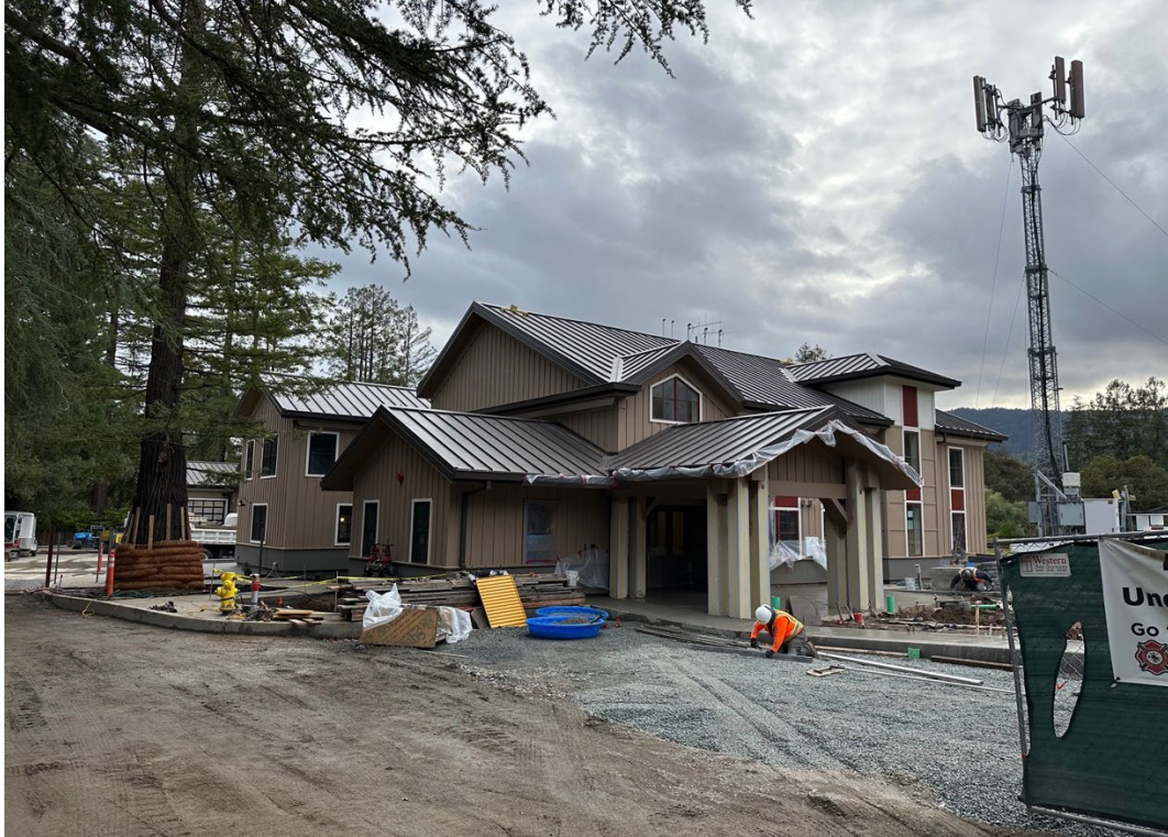
Preparation for east driveway with grading and base rock
