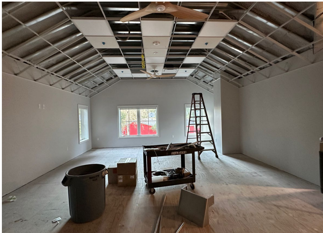
Drop ceiling installation in second floor gym
