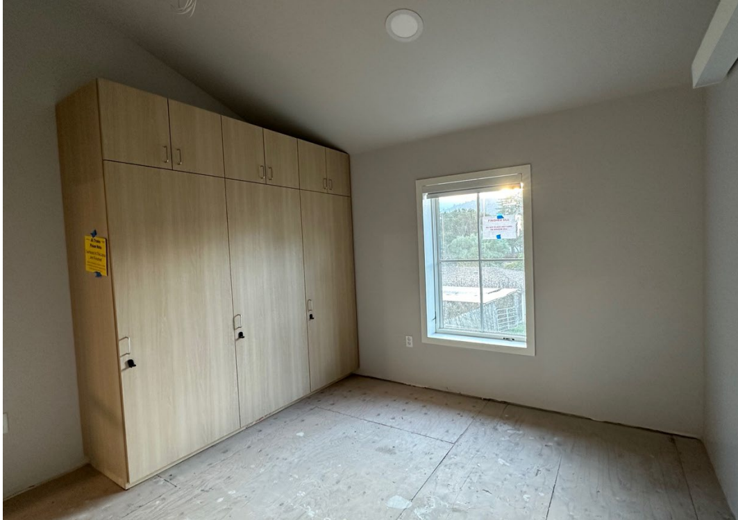
Bedroom casework (lockers) complete
