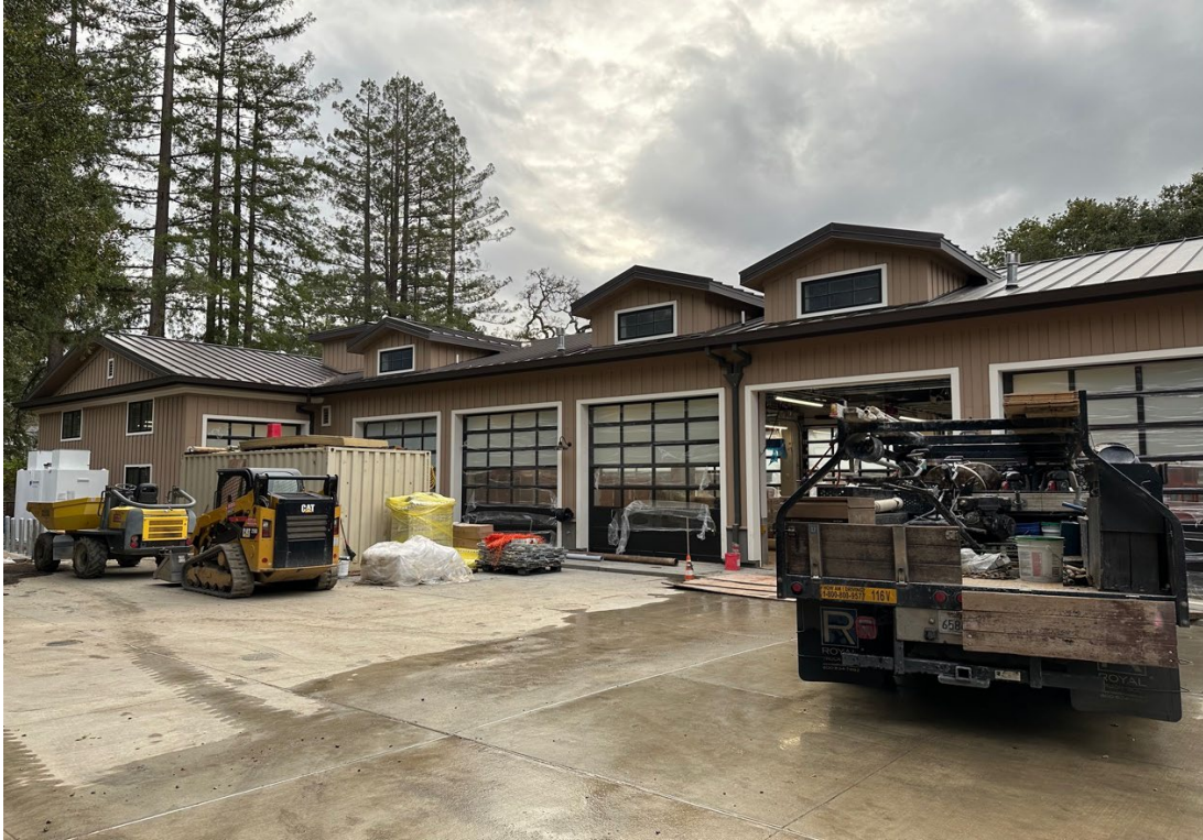
East apparatus bay concrete pad complete
