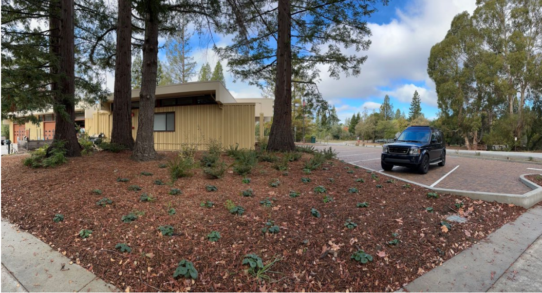
South driveway landscaping complete, front parking lot complete with paint striping.
