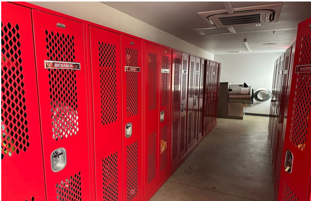
New station 8 turnout locker room with extractor
