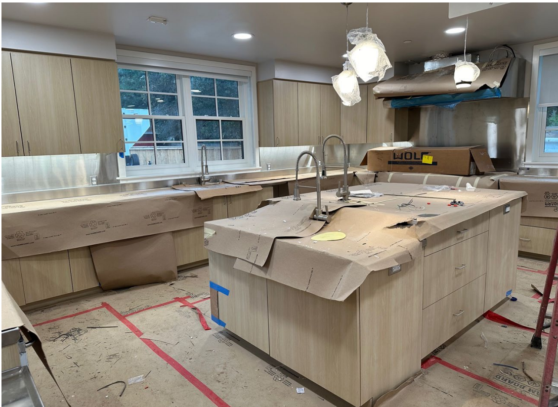
Kitchen casework complete, fixtures installed and range & hood installation underway
